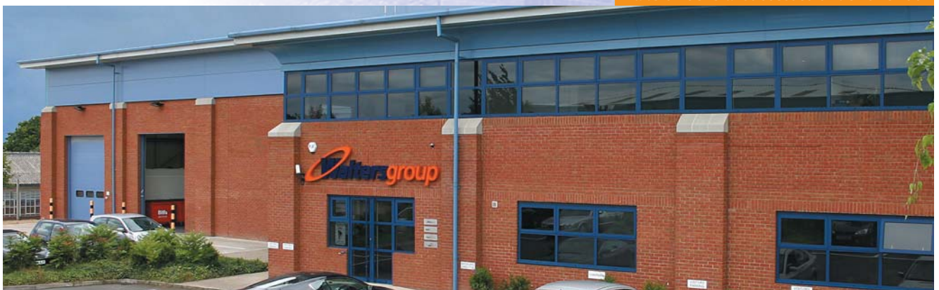
The Walters Group - Head Office & Manufacturing Centre of Excellence in High Wycombe
